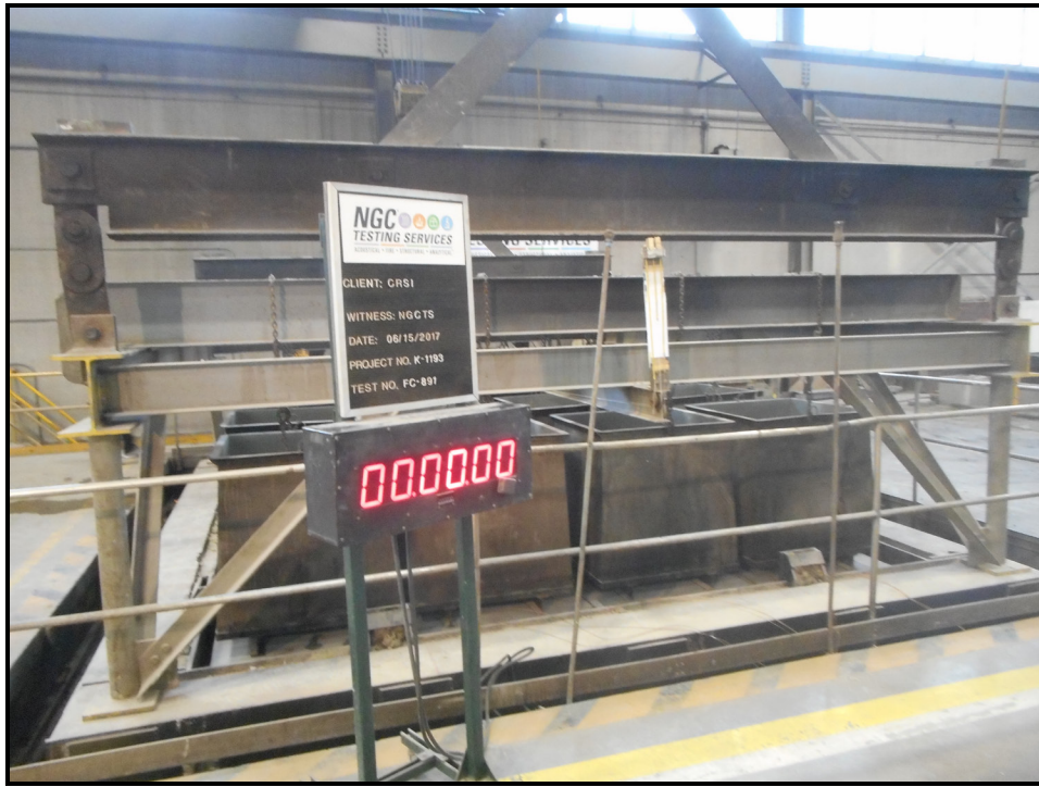
Unexposed Side – Start of Fire Endurance Test
