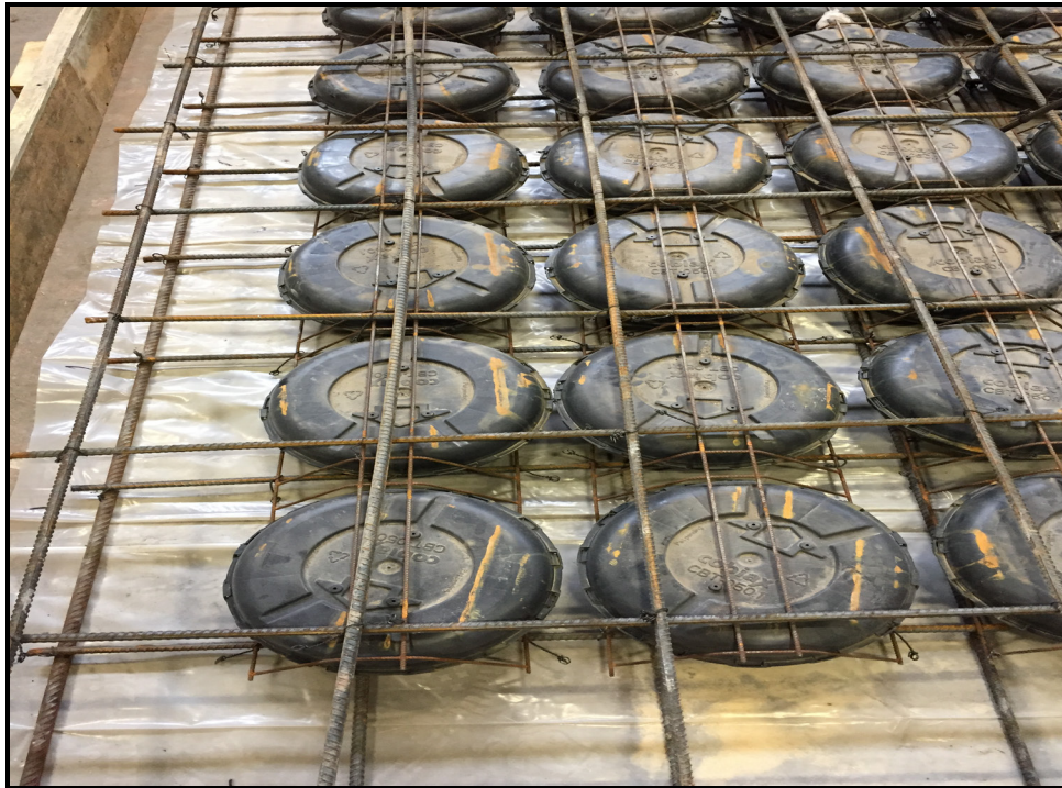
Test Specimen Construction – Close-up of Plastic Voids and Rebar Layout
