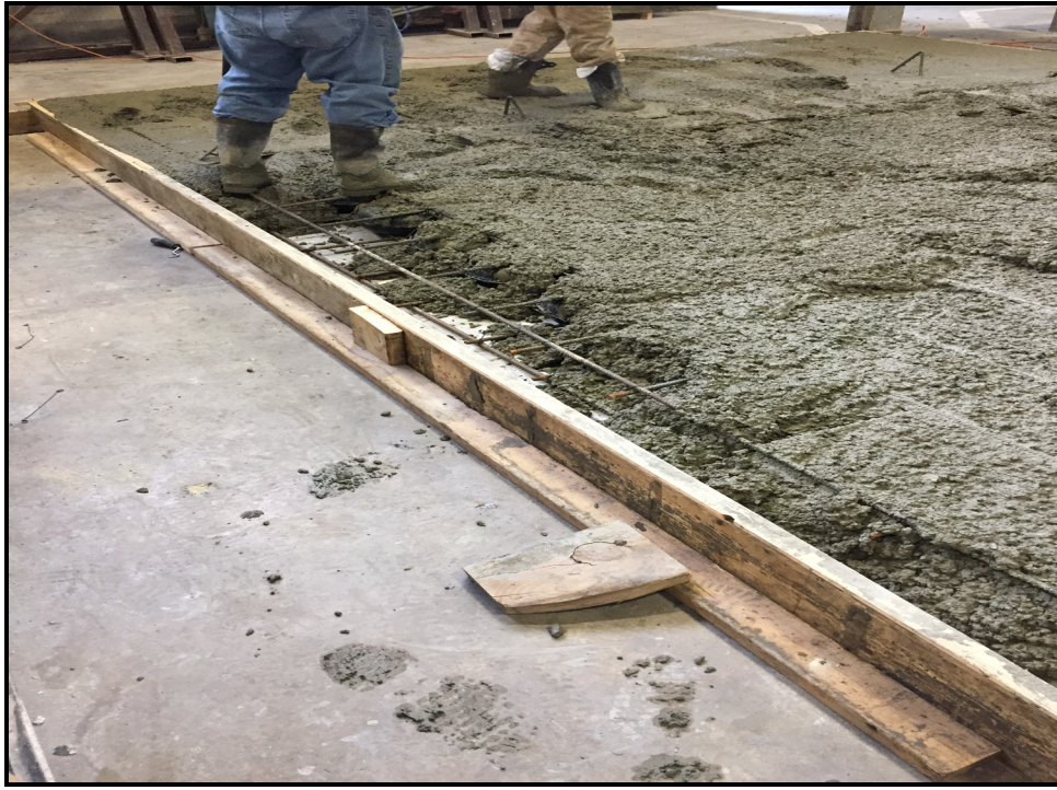
Test Specimen Construction – Pouring Concrete Slab
