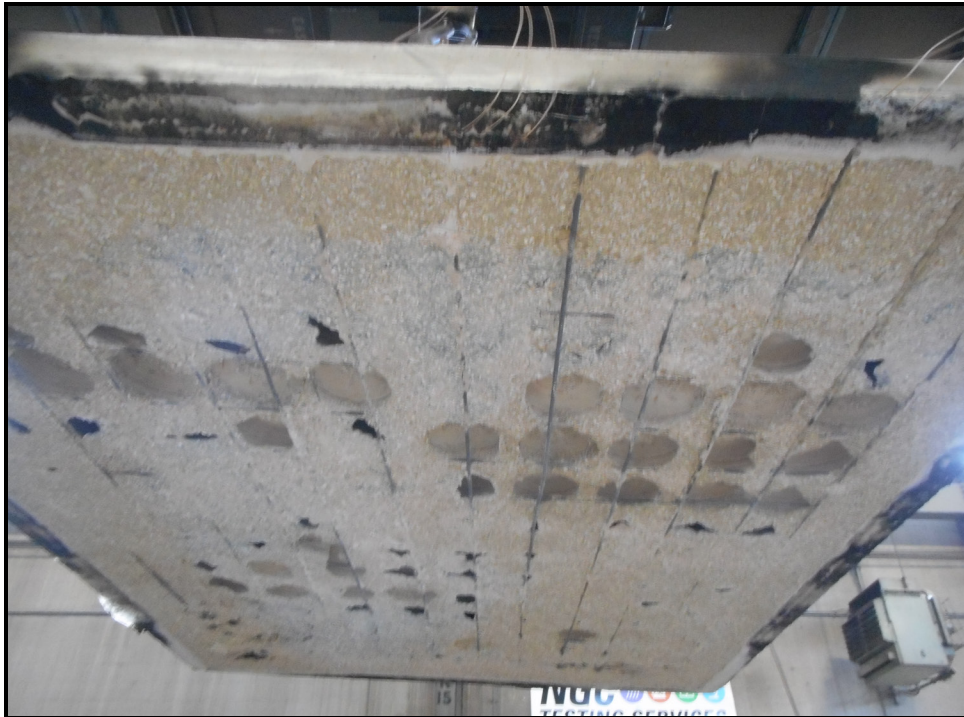
Exposed Side – Post-Test (Slab Cooled for 24 Hrs.)
