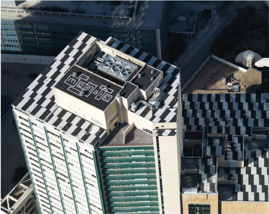
Low-slope roofing membrane self-adhered with primer application and consisting of a SBS-modified bitumen cap sheet and base sheet.
