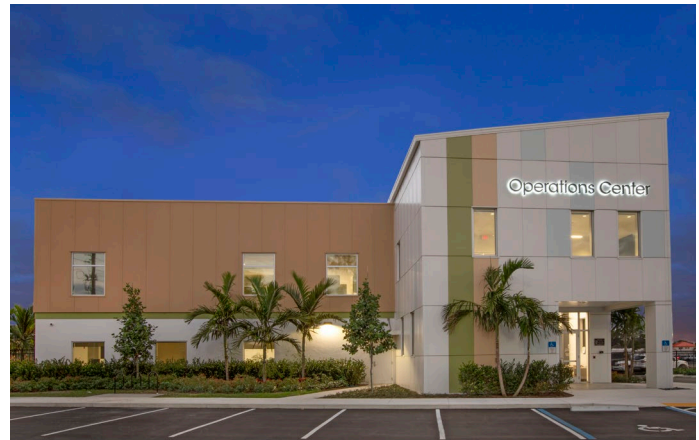
Figure 2: Palm Beach Gardens Emergency Operations Center
