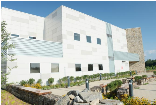
Figure 1: Loudoun Water Treatment Facility
