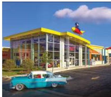
Metal is used for coping, trim and similar functions other than cladding roofs and walls, like on this fueling station in Illinois.
