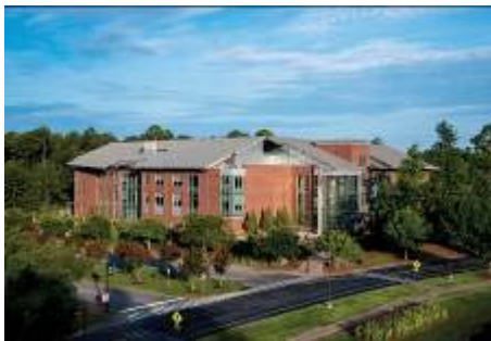
Higher education facilities are commonly roofed with metal panels, as seen here on a science building in Georgia.
