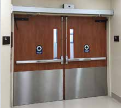
Pair—side load lintel mounted header
