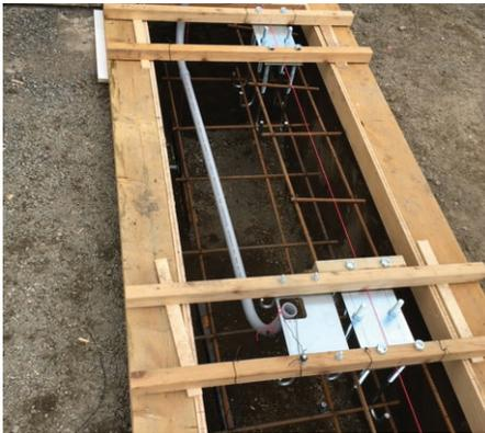
Line up the bolts. Use a string line, template, or other means to ensure bolts are correctly spaced apart. Use the (I) dimension from the project summary. Line up with the other carriage and run parallel to the gate opening.
